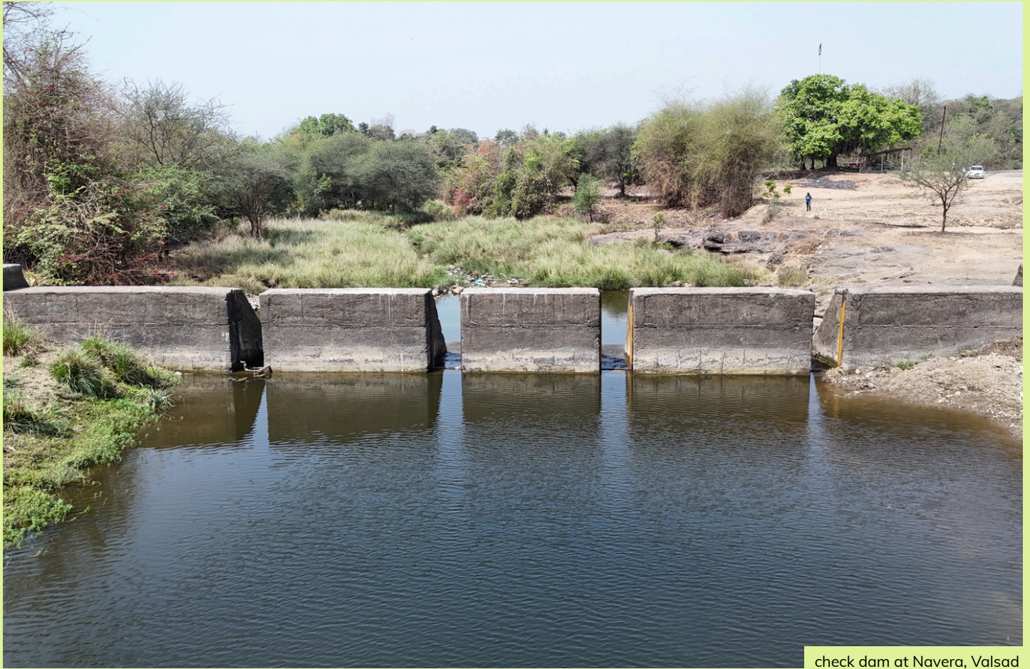
check dam at Navera, Valsad
