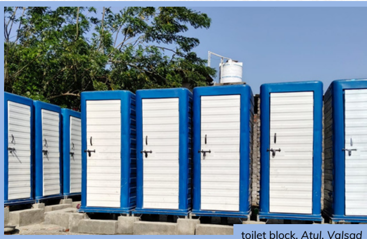
toilet block, Atul, Valsad
